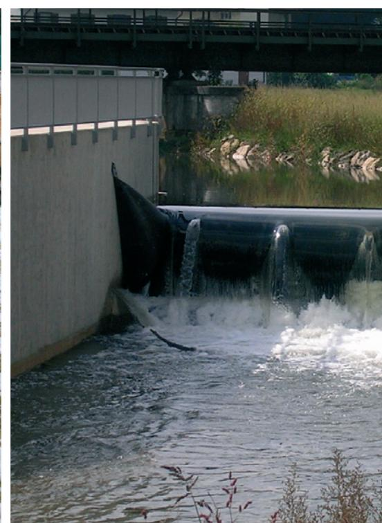
The number of **Arcon AquaPro** Rubber Dam installations is growing all the time as more engineers move away from conventional steel gate dams to flexible, safer and more reliable rubber dam systems. This trend can be seen from the rapidly increasing number of installations worldwide.
